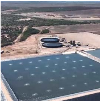
Aeration and Chemical Injection
