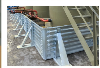
Steel Wall/Spray Liner Containment Systems
