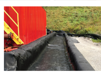
Secondary Containment HDPE Liner Systems
