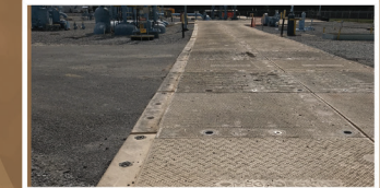
COMPOSITE MAT RENTAL AND INSTALLATION FOR SITE ACCESS
