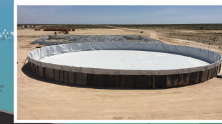
ABOVE GROUND STORAGE TANK (AST) INSTALLATION AND RENTAL
