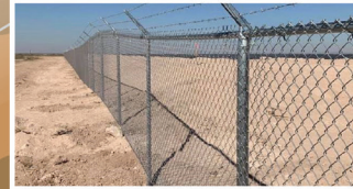
FENCING AND ADDITIONAL SITE SERVICES
