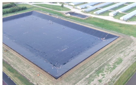
RNG Containment, OK
