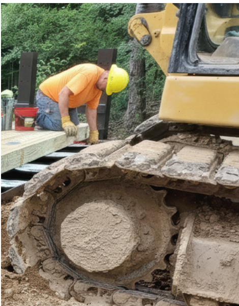
Installing clips facing end plate on first deck panel.
