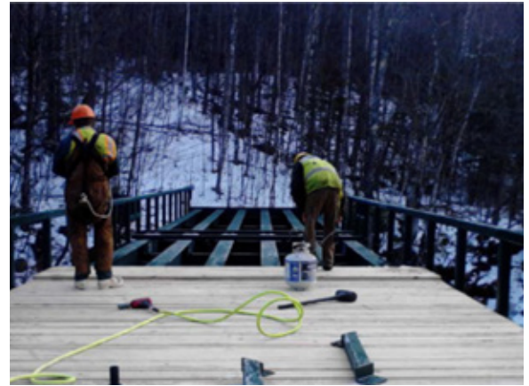
Installing timber deck
