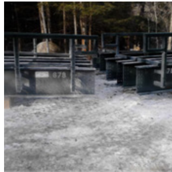
Six [two-beam] partial-length sections offloaded and awaiting splicing
