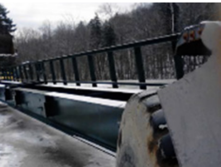
Carrying full-length section from staging area to crossing with two loaders
