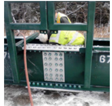
Splicing [bolting] two partial-length sections
