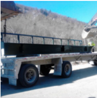
Offloading partial-length section with loader/excavator
