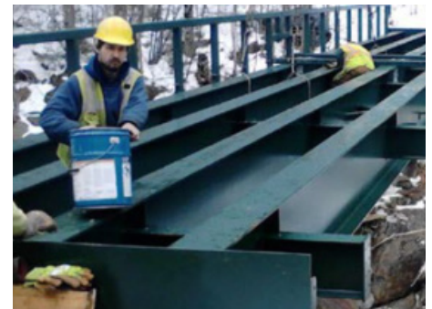
Bolting first and second full-length sections together
