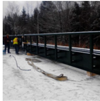
Splicing [bolting] two partial-length sections together
