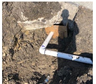
Liner installed under the drainage system to capture water flowing under the pond.
