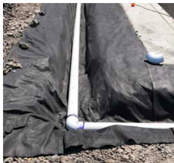
Piping installed through the kettle and into the drainage system.
