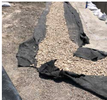
River rock was installed in the trench to help collect water and guide it to the underdrain.
