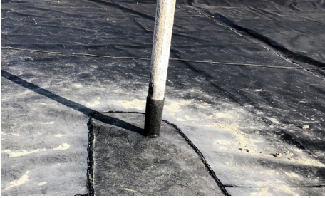
Pipe protrusion fitted with a boot to add strength to the liner
