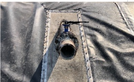
Batten bar used to attach liner to the concrete boot.
