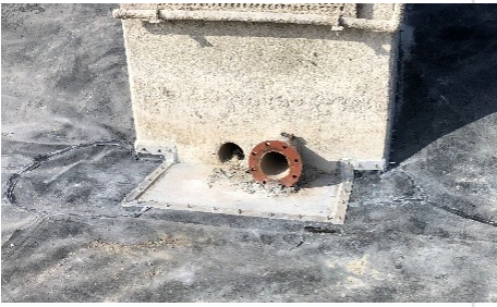
Liner carefully cut to fit and attached to concrete islands with batten bar
