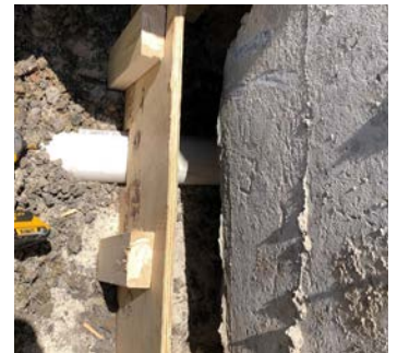
Concrete kettles drilled to enable installation of the pipe into the kettle.
