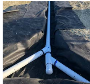
Perforated PVC pipe installed underneath the pond.
